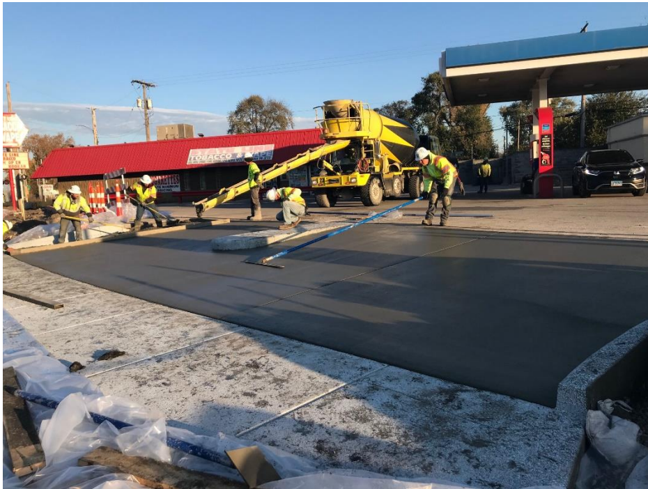
Figure 2: Milestone pours drive way near State Line
