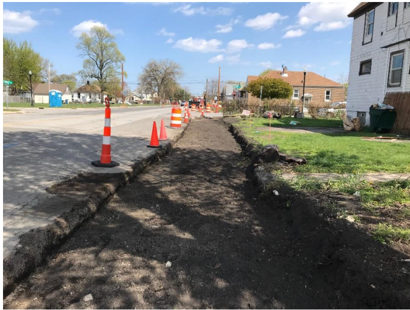
Figure 1: Milestone Removed Sidewalk
