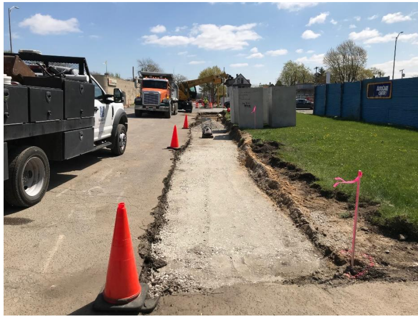
Figure 2: Milestone Placed Compacted Aggregate for Temp HMA
