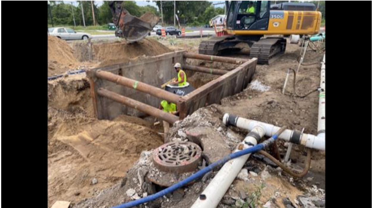
Figure 1: Installing Sanitary Sewer
