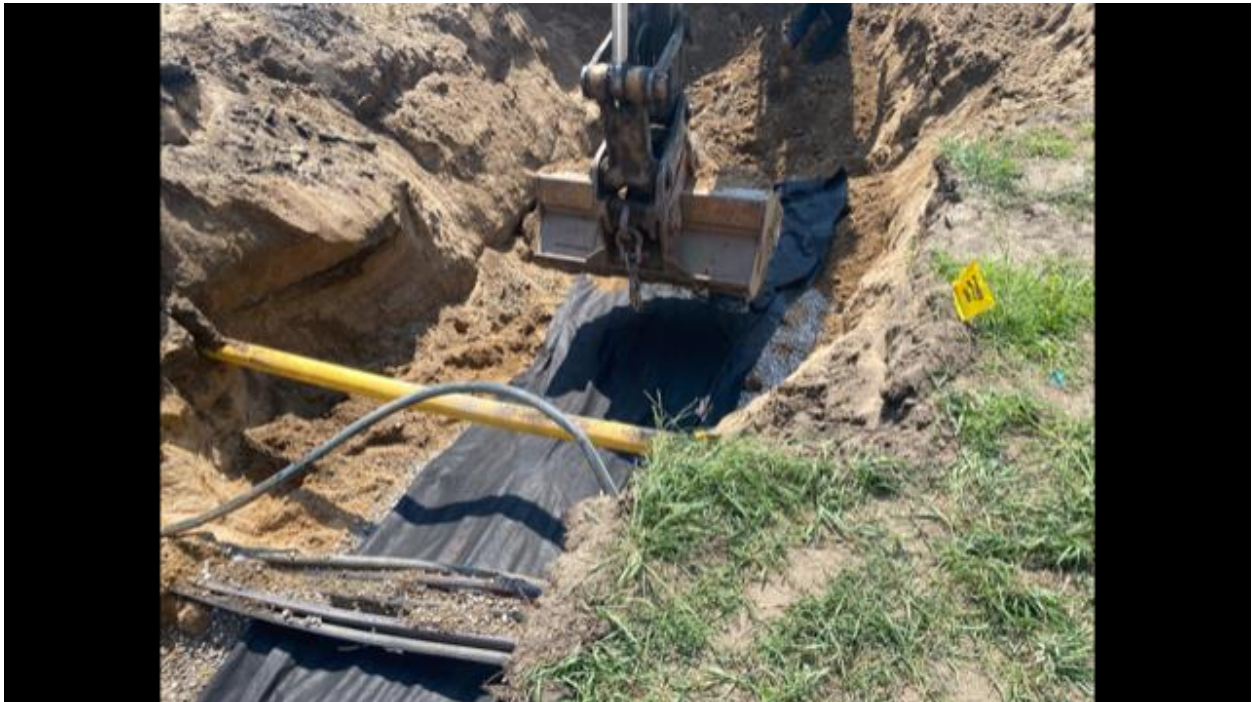
Figure #2: Installing Sanitary Sewer Laterals with Geotextiles
