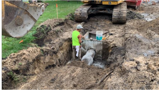
Figure 2: Grimmer installs an Inlet
