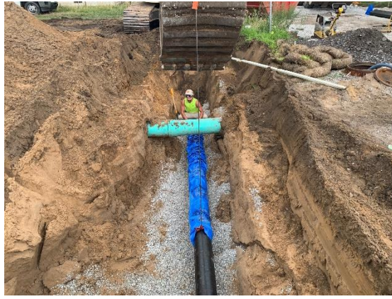
Figure 1: Grimmer installs Watermain
