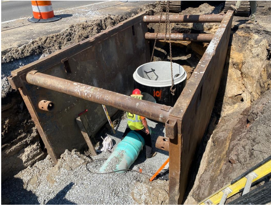
Figure 1: Installing Sanitary Sewer
