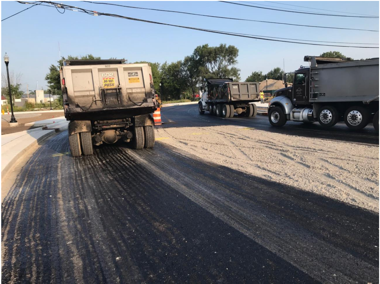
Figure 1: Asphalt Trucks Line Up for Paving
