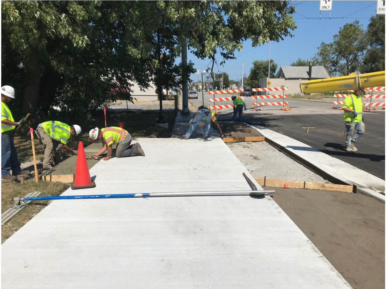
Figure 1: Milestone pouring driveway on Hohman
