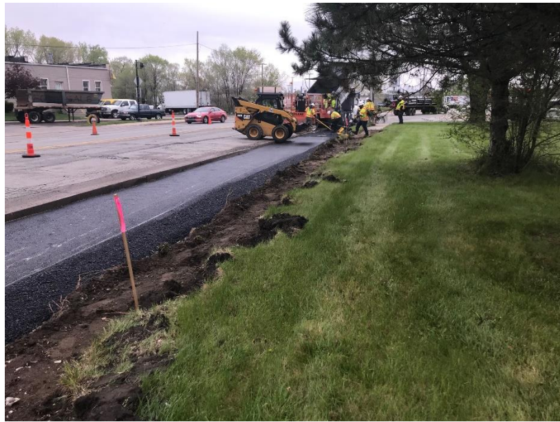
Figure 2: Milestone Paves Temp Road Near Baltimore
