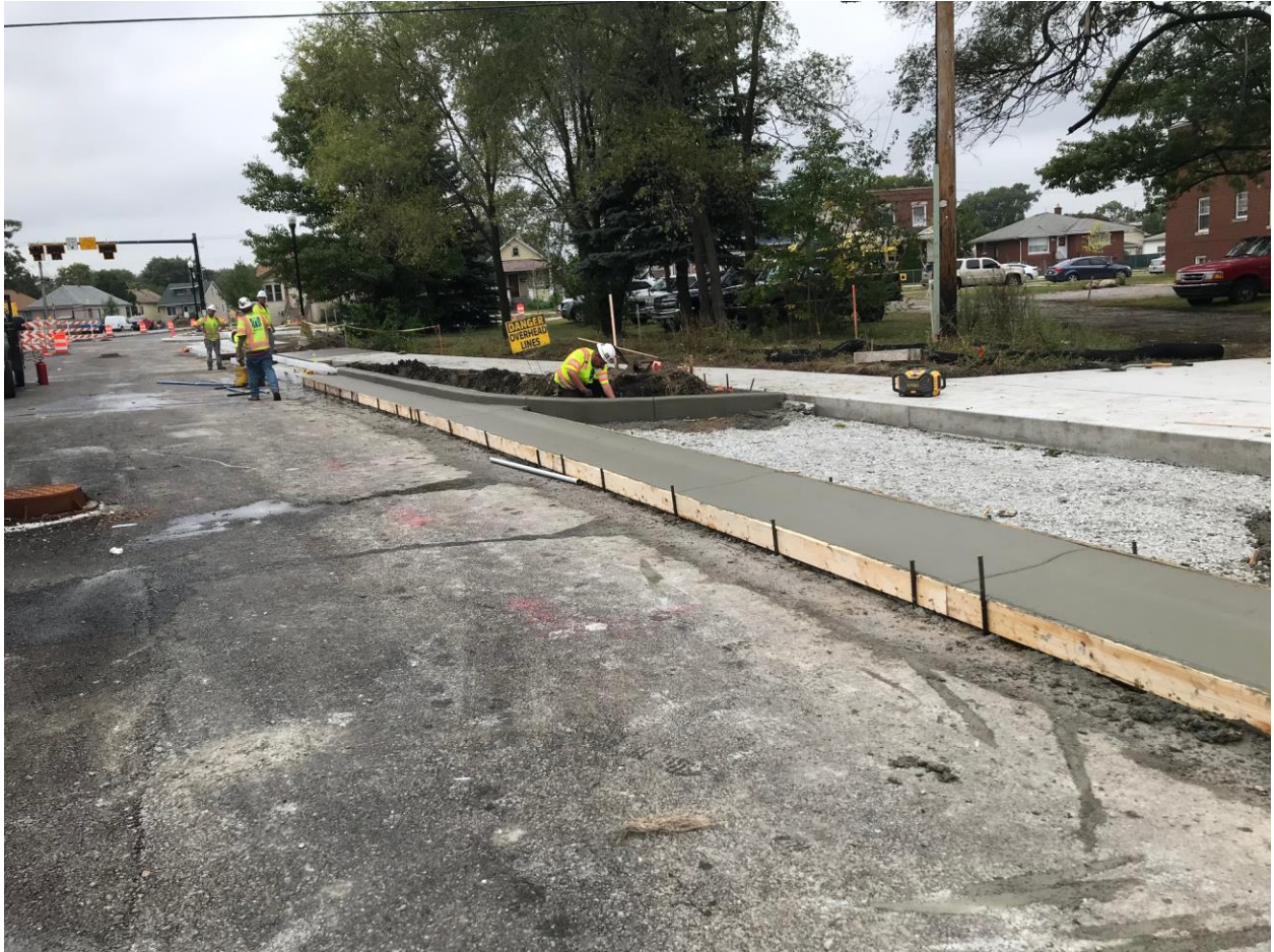
Figure 1: Milestone poured curb and gutter East of Torrence
