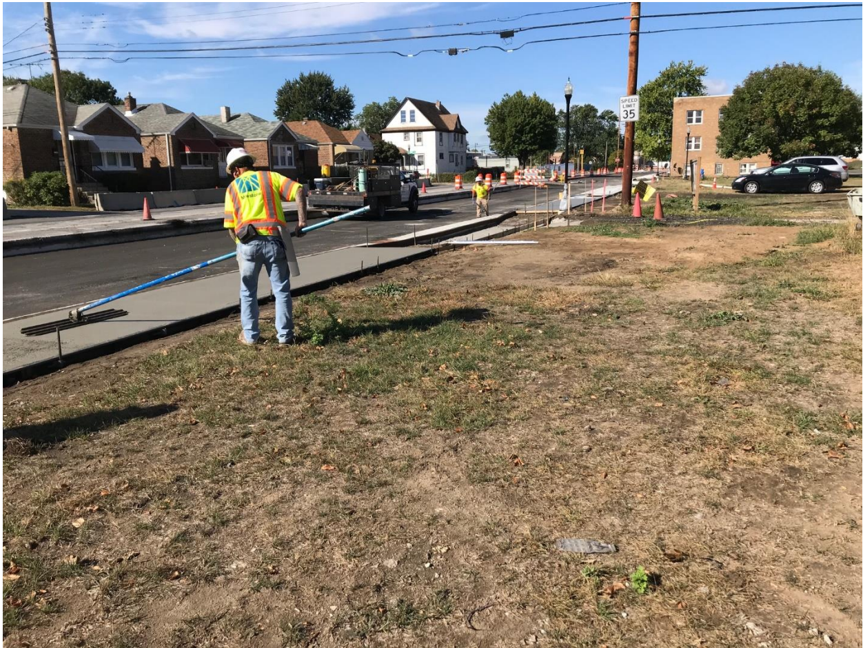
Figure 1: Milestone pouring Sidewalk between Cameron and Johnson
