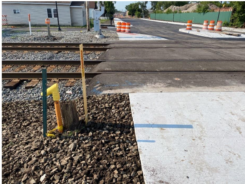
Figure 2: Finishing touches at CSX
