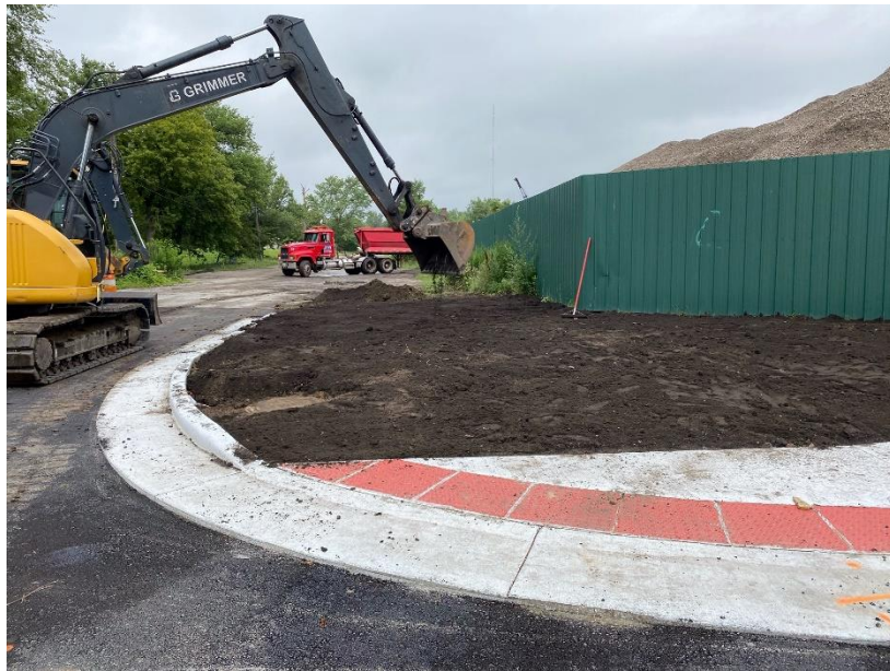
Figure 1: Topsoil being placed at Marble
