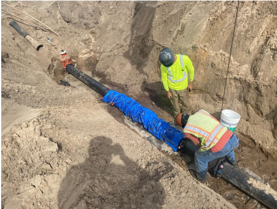
Figure 1: Grimmer finishing water main connections
