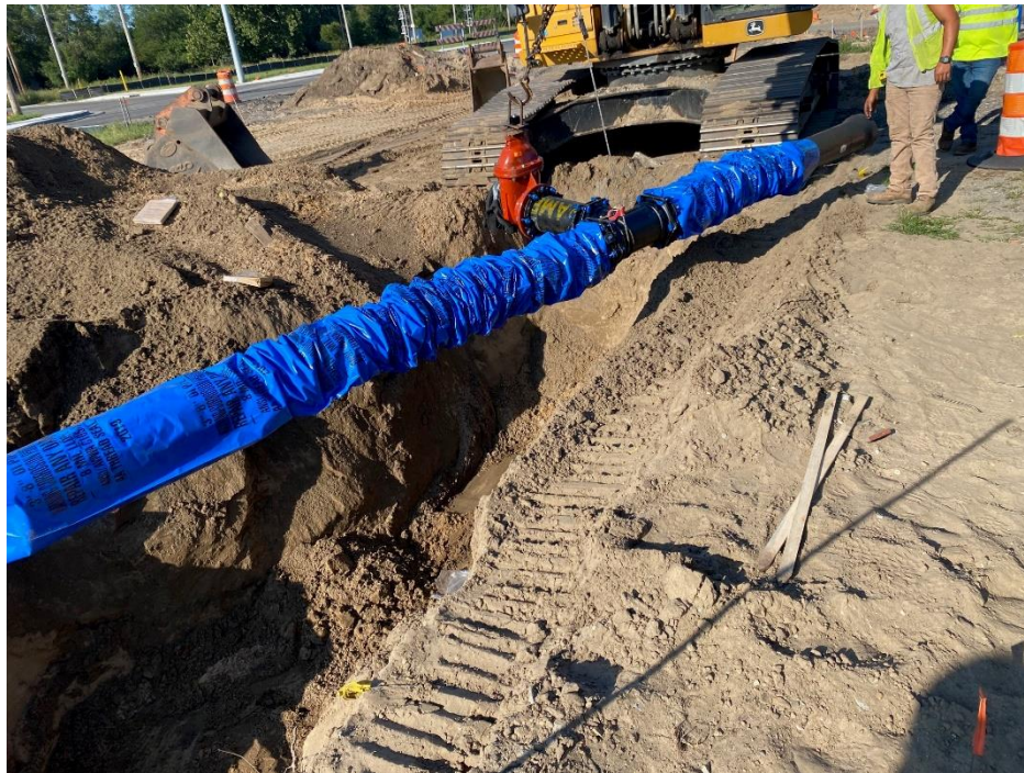
Figure 1: Installing Water Main and Valve
