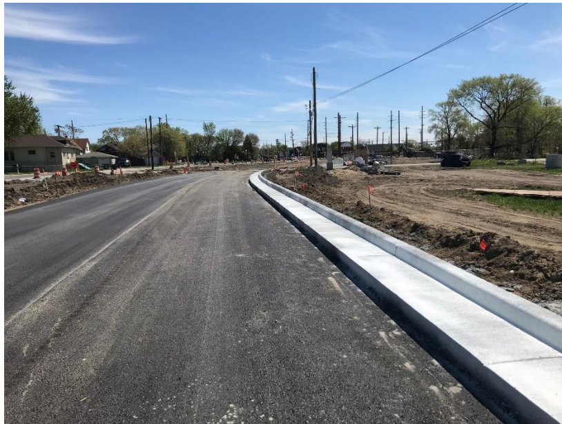
Figure 2: New Curb and Gutter Installed on Gostlin
