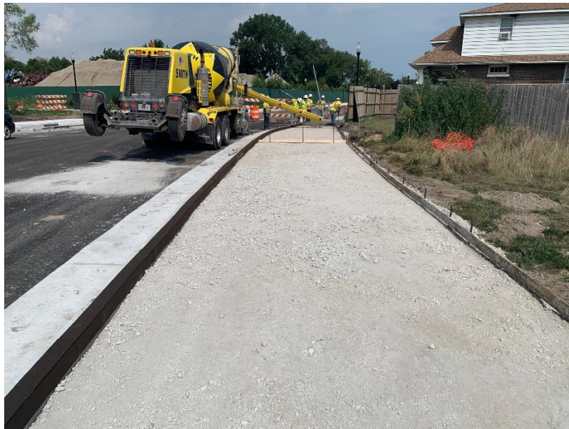
Figure 22: Multi-Use Path Being Poured
