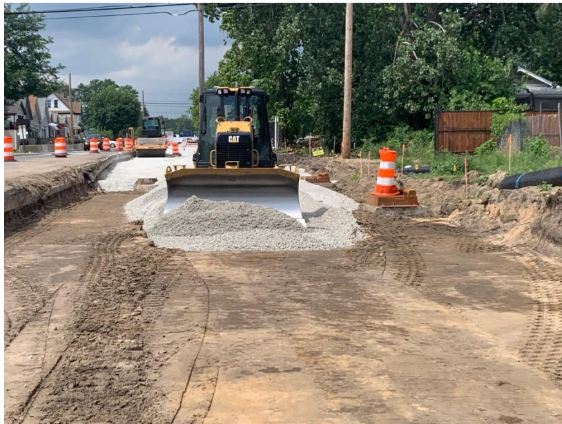
Figure 1: Subgrade Treatment Installation
