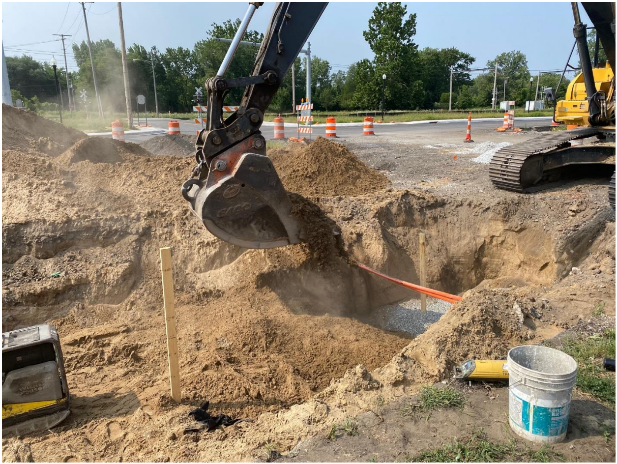
Figure 1: Installing Sanitary Sewer near Gostlin/Dearborn
