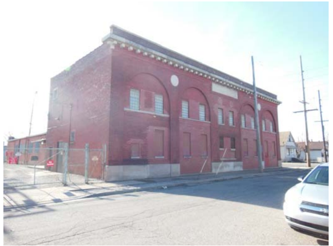
40044_Sheffield and Hanover_4533 Sheffield north elevation.JPG
