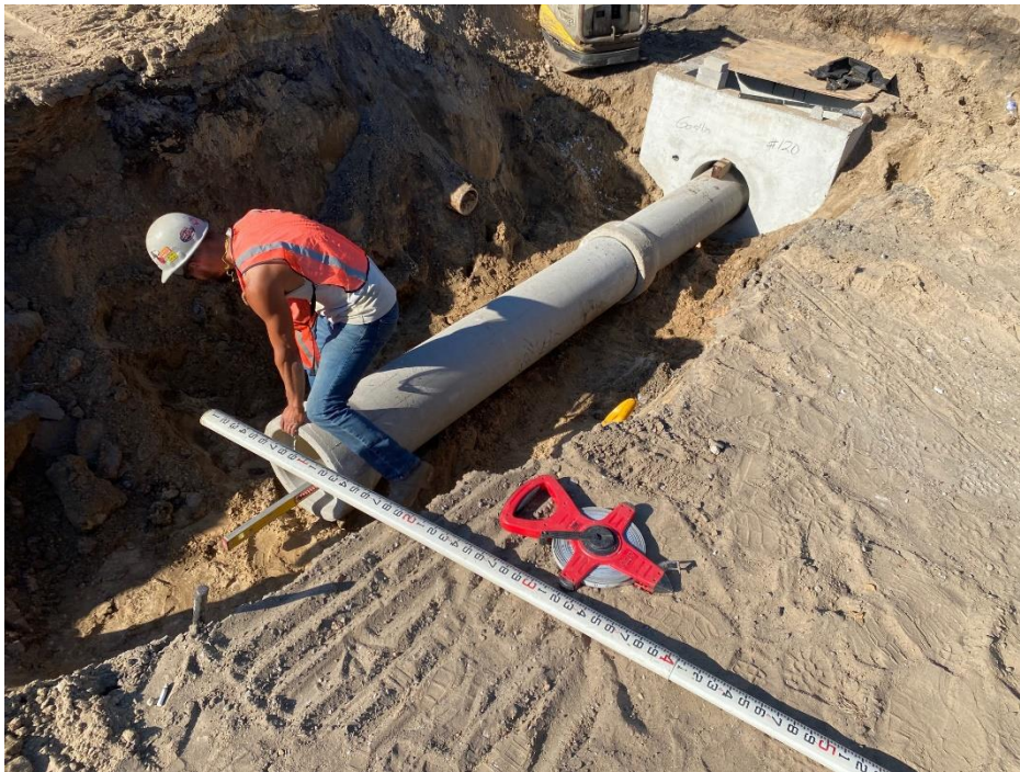
Figure 1: Installing Storm laterals
