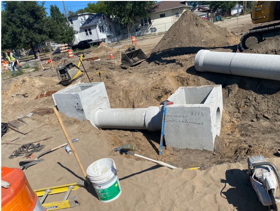
Figure #2: Storm Sewer along Gostlin
