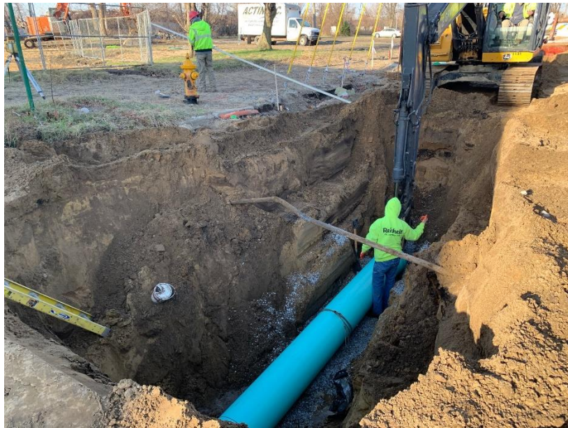
Figure 2: Hanover Storm Sewer
