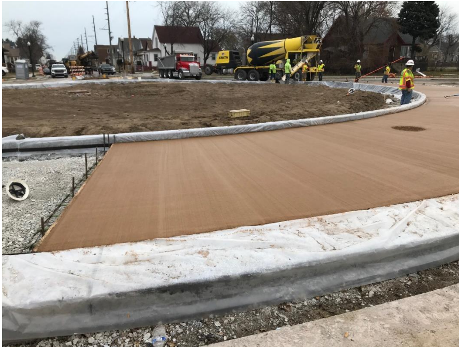
Figure 1: Milestone pours colored concrete for the roundabout truck apron
