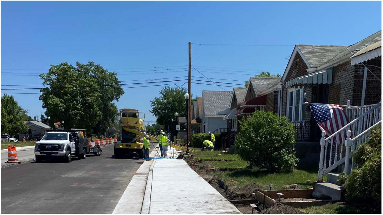
Milestone pouring sidewalks for houses.
