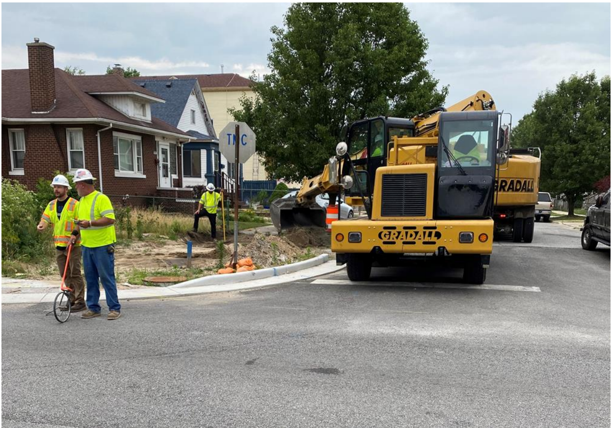
Milestone grading for tie-in on Henry.
