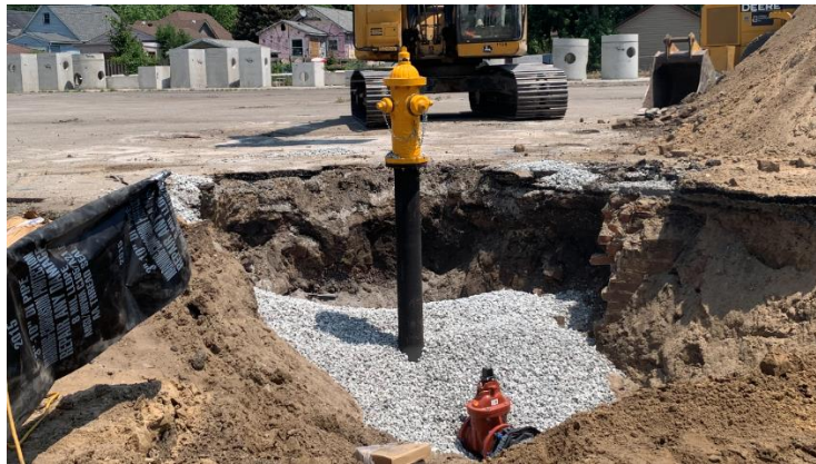
Figure 2: Grimmer installs new fire hydrant
