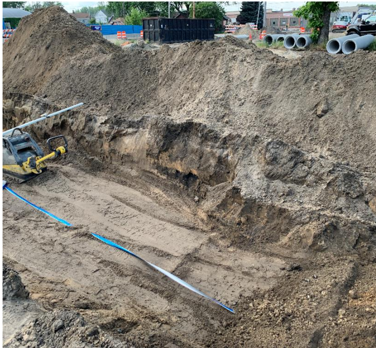
Figure 1: Grimmer places tracer tape above new water main
