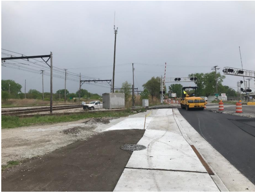
Figure 1: Milestone rolling Intermediate HMA at State Line
