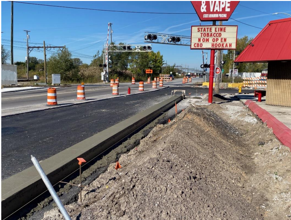
Figure 2: Curb and Gutter placed at State Line
