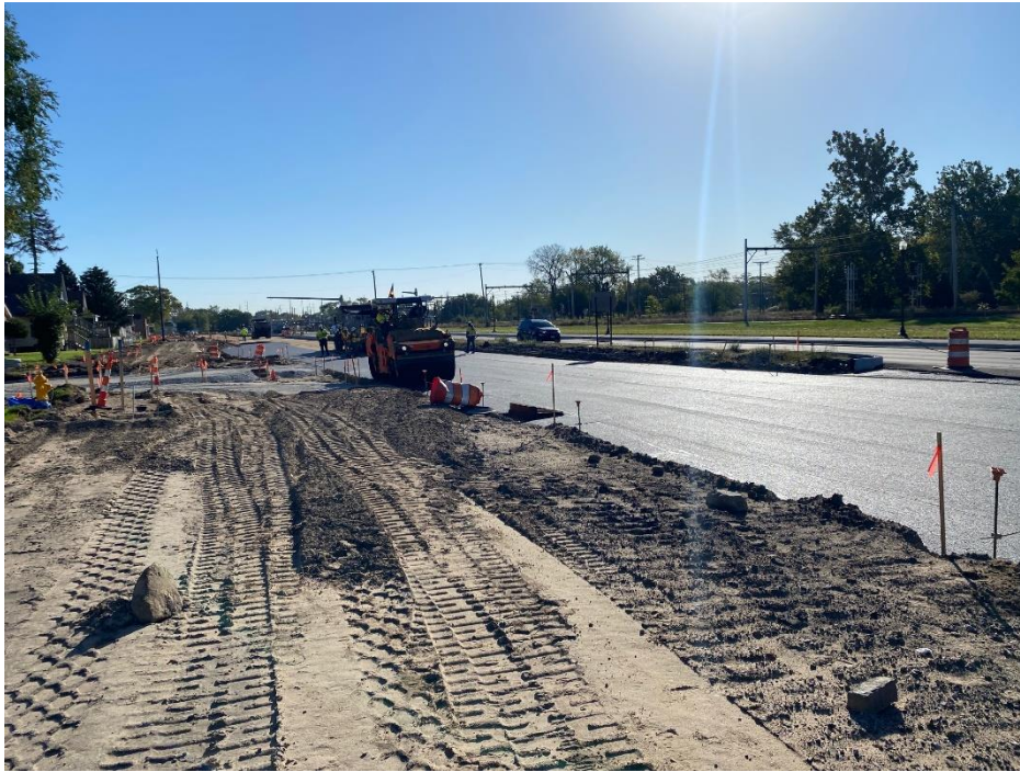
Figure 1: Base HMA is rolled
