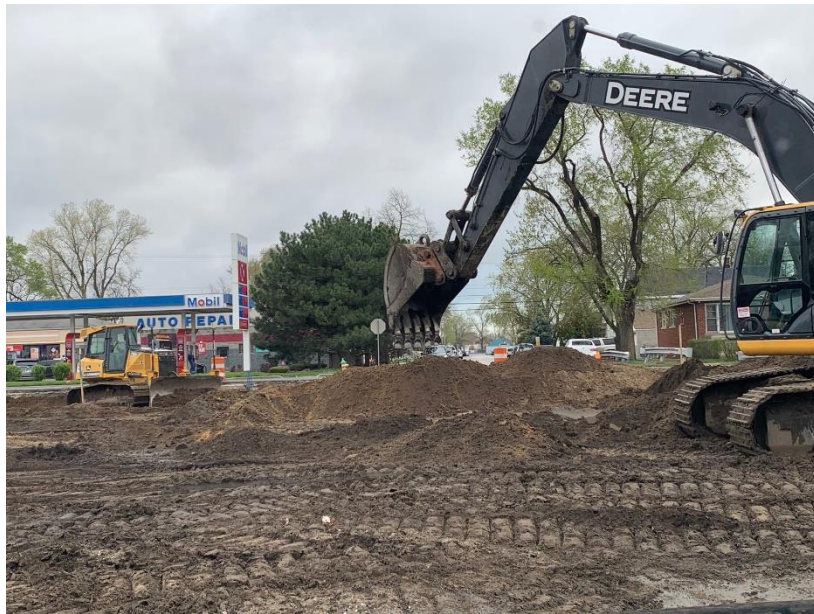
Figure 1: Grading Efforts Near State Line
