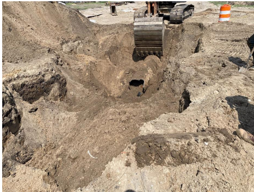
Figure 2: Old Watermain Being Removed from Sheffield
