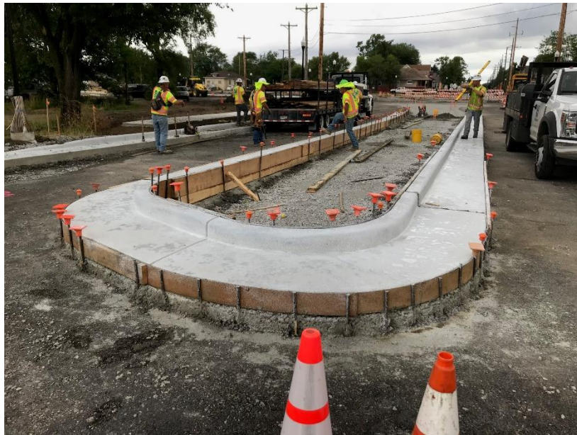
Figure 1: Sheffield/NICTD Crossing looking North
