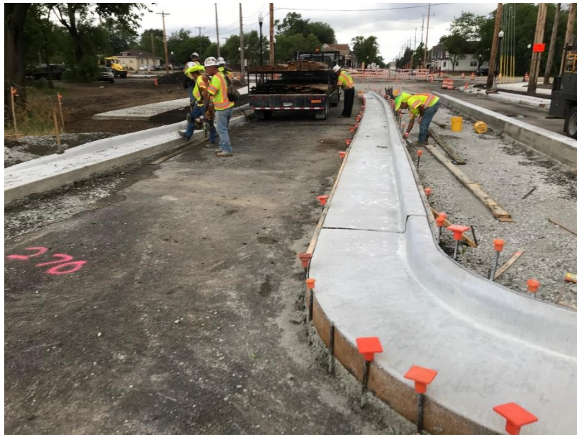
Figure 2: Southern approach of Roundabout Looking North
