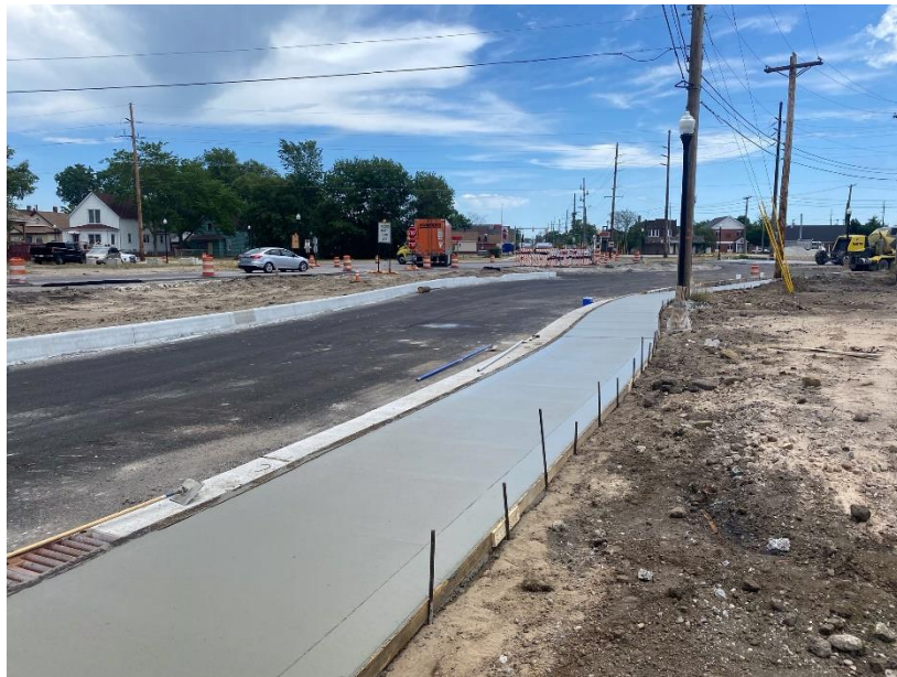
Figure 1: Sidewalk west of Sheffield looking East
